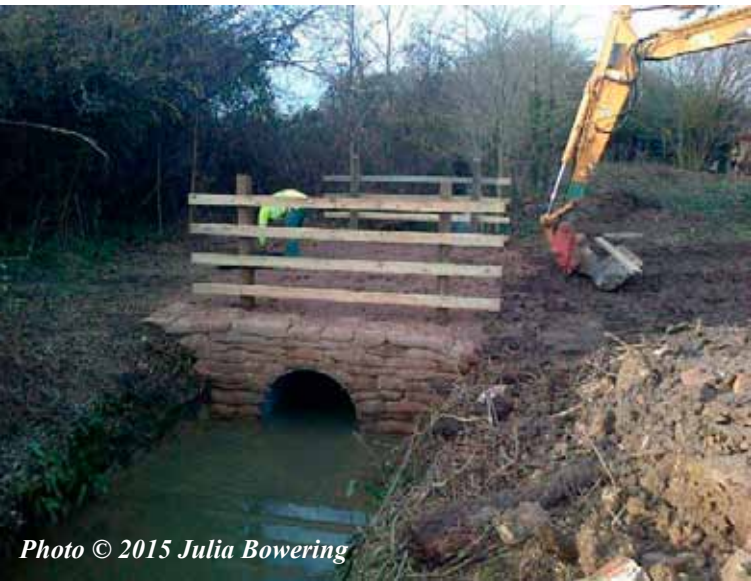
New culvert in Almodington
