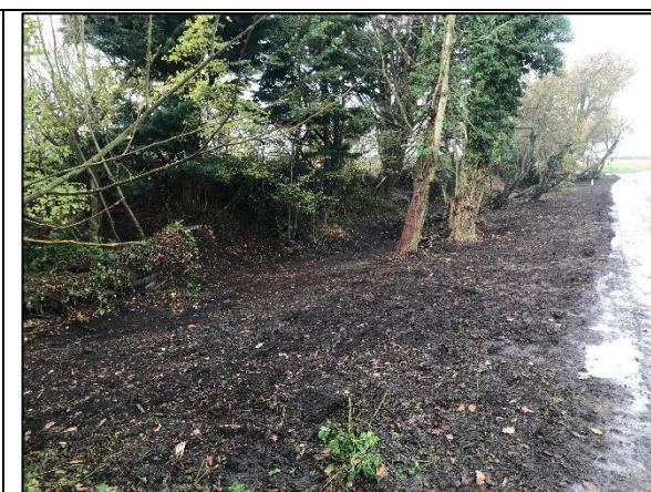
The Elms ditch - This is a large wide ditch full of broken-down old trees, debris from previous trees falling, bramble and undergrowth. This area frequently floods, so by digging the ditch out and increasing its' capacity, it will be able to tank more water. This corner ditch when opened up and light let in will host more diverse vegetation. A grip off the road has taken water into the ditch to help reduce road flooding.
