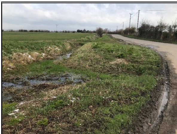
Corner pond / ditch area opposite The Elms – A junction area just before a culvert that carries water underneath the road. This was a large pond on the verge corner and had slowly been filled in. By reinstating it as a pond again with a grip off the road, this has helped with flooding on this road junction.
