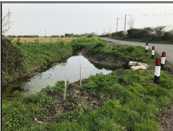
Corner pond / ditch area opposite The Elms – A junction area just before a culvert that carries water underneath the road. This was a large pond on the verge corner and had slowly been filled in. By reinstating it as a pond again with a grip off the road, this has helped with flooding on this road junction.
