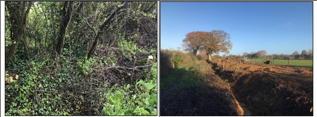
Sidlesham Common Ditches – ditches recovered to re-join the wetland system to the network and reduce the groundwater levels
