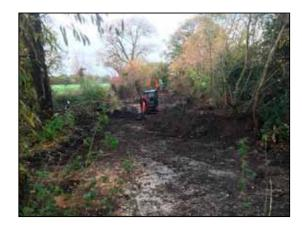
A contractor with a digger was brought onsite to dig out this wetland areas. The spoil was to be left onsite and curving banks created. A deeper base has been created to hold water for longer during the year.
