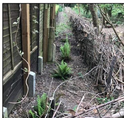
Dead hedge along the edge of a site – using chestnut stakes to hold the slotted material in place.
